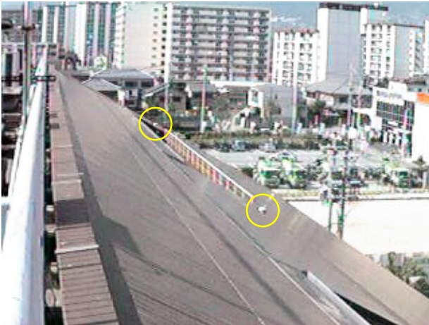
Figure 3. Antenna installation on the roof
